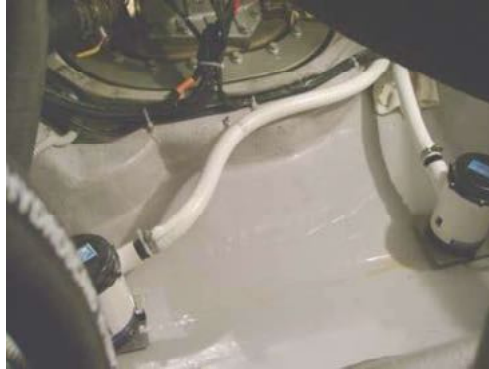
FIG. 4.14-2 – bilge pump position inside engine room
